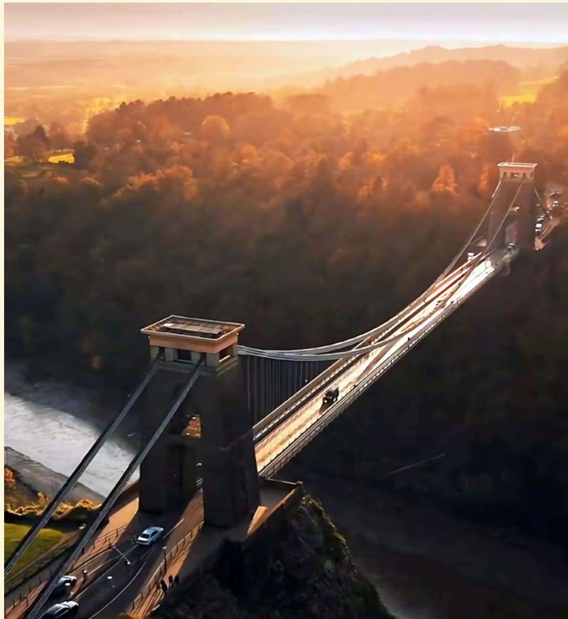
Clifton Suspension Bridge
